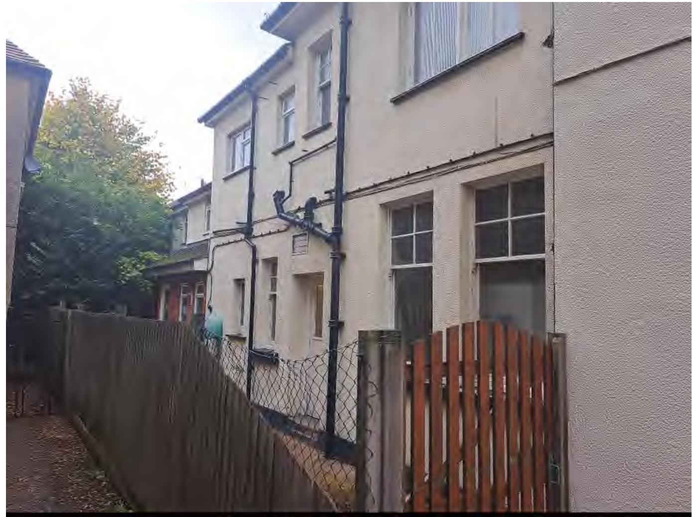
Flank elevation of 9 Imperial Avenue
